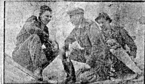
Roof-top discussion between Maurice Thow (left), the village electrician; Alf Evans (centre), the village joiner, and Alf's son Jack.
